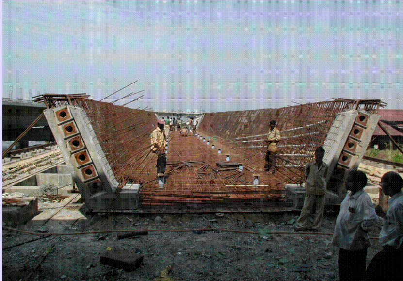
Figure 4-6.14 Fabrication of reinforcement (Courtesy: Cochin Port Trust, Kerala)
