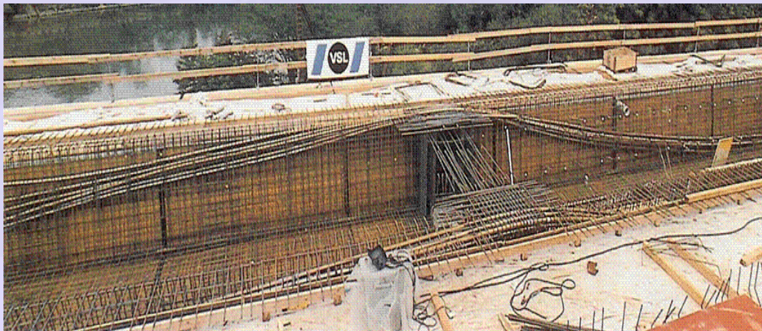
Figure 4-6.5 Tendon profiles in a continuous bridge girder
